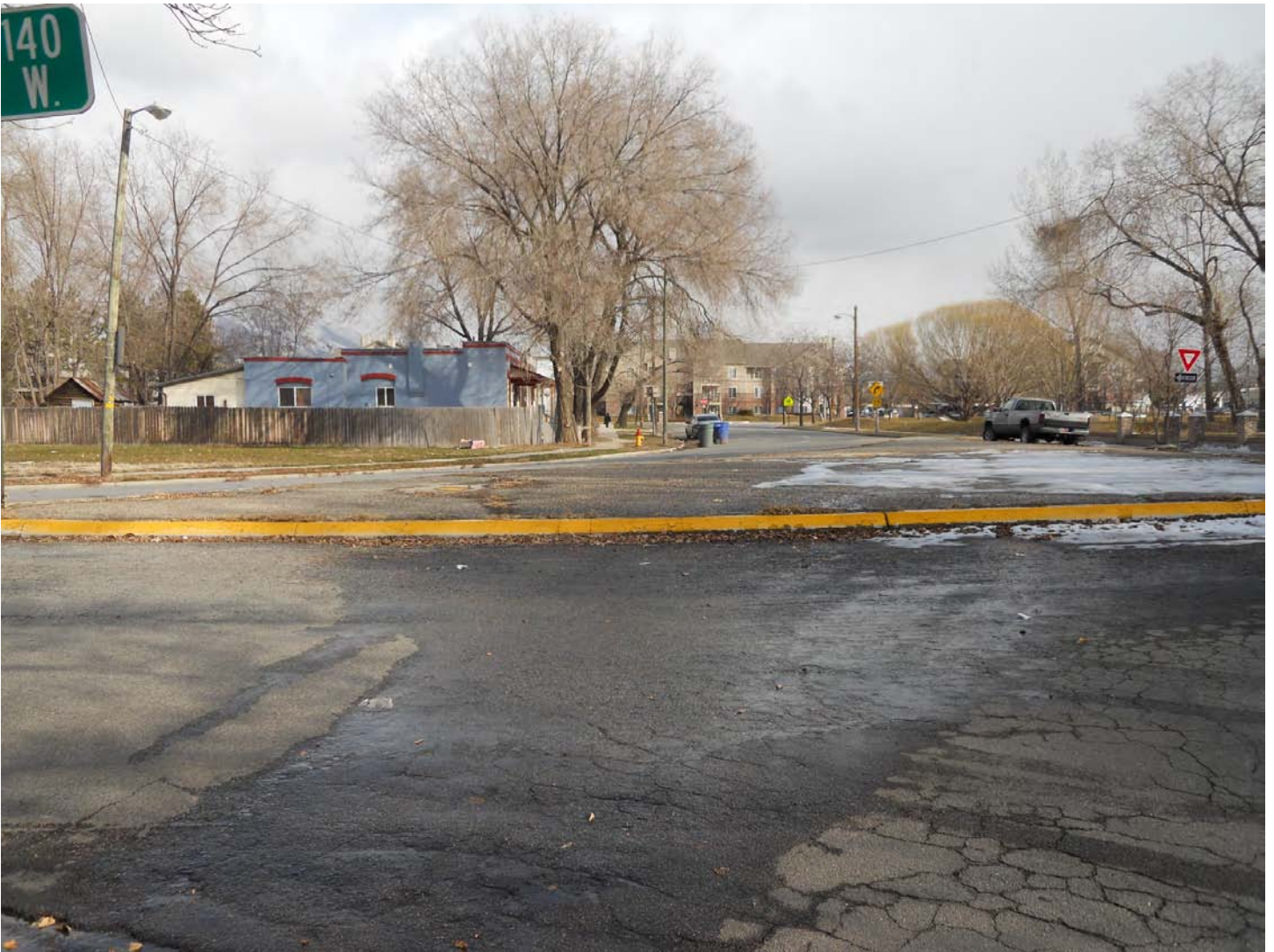
This photograph is looking towards the east along Goltz Avenue. Jefferson Street is on the left side of the photograph and curves to become Goltz Avenue. The Jefferson School Apartments can be seen in the background. That property is zoned as R-MU.
